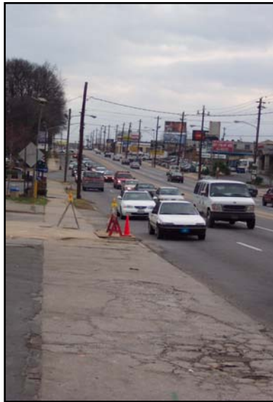
Broken sidewalks at Northside/14th Street
